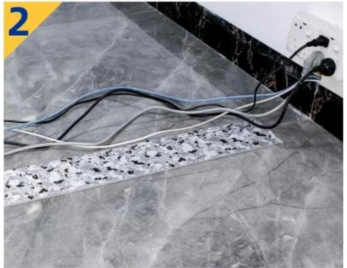
2 Attach to the location where the wires need to be placed, and press the tape to stick firmly.
