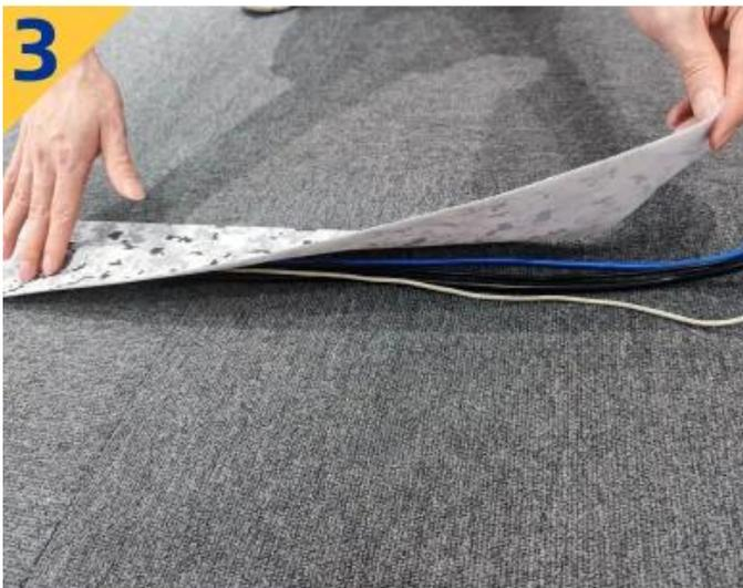
3 After arranging the wires neatly, close the covers by attaching hook to carpet.
