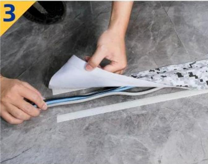
3 Open the cable cover by tearing off one of the hook side and put the wires inside.
